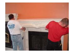
Make sure that side of legs and header are well aligned.
