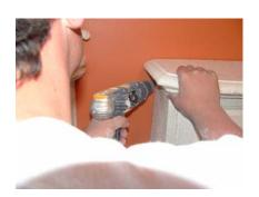
At both ends of the header, find studs behind the wall and drill holes at a 45 degree angle from the header to the wall (facing studs). Screw the header to the wall using ordinary wood screws (3" or 4", #10). Repeat operation to the side of header clearing the mantel shelf.
