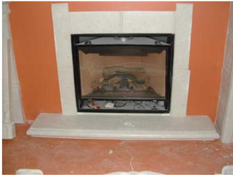
Level the podium (hearth) with the floor using brick mortar or thinset masonry mix (not included). This stage should be taken seriously to obtain a successful assembly.
