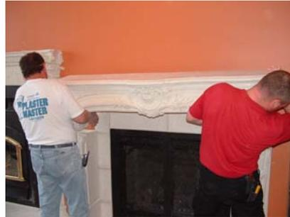
Make sure that side of legs and header are well aligned.
