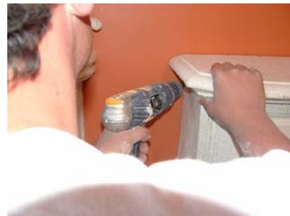
At both ends of the header, find studs behind the wall and drill holes at a 45 degree angle from the header to the wall (facing studs). Screw the header to the wall using ordinary wood screws (3" or 4", #10). Repeat operation to the side of header clearing the mantel shelf.
